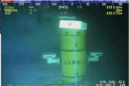
ROV (remote operating vehicle) captures the moment Samo-1 is spudded
